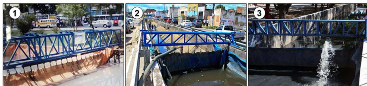
Figure 1. Examples of mobile dams: 1 - installed on the Derby/Tacaruna channel in Recife - PE; 2 - installed in the channel Avenida Airton Teles in Aracaju - SE; and 3 - installed on the Gulandi channel in Maceió - AL. Source: (Hidromax Construções, 2003; Rodrigues, 2017; SECOM and Antônio, 2014).
