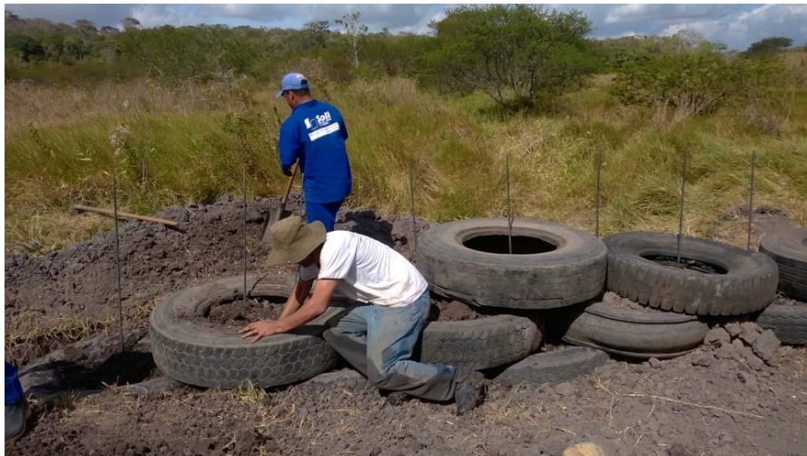
Figure 16 - Assembly of the fourth layer of tires. Source: Vasconcelos (2016).
