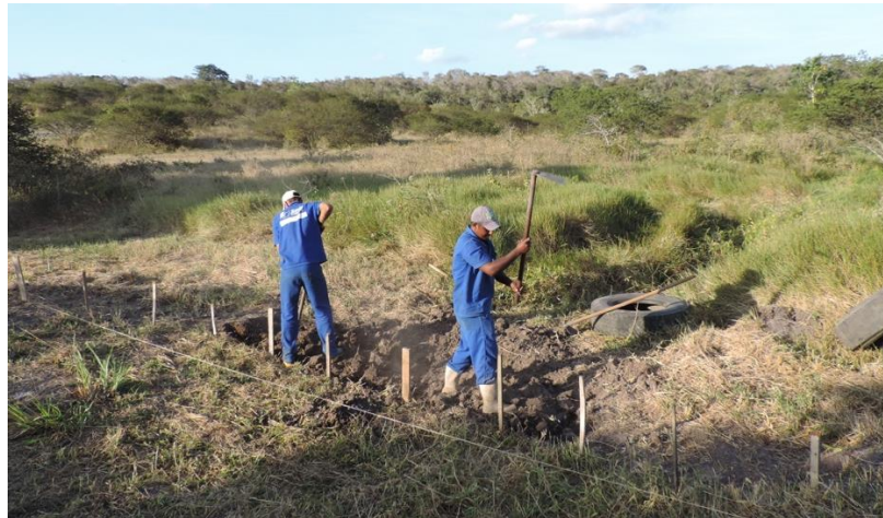
Figure 12 - Opening of the trench for placement of the first layer of tires. Source: Vasconcelos (2016).
