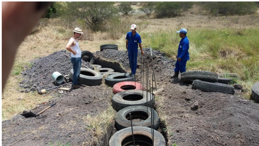
Figure 14 - Assembly of the second layer of tires. Source: Vasconcelos (2016).
