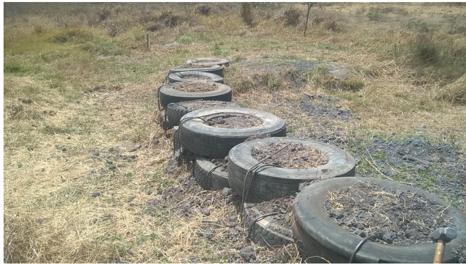
Figure 19 - Barrier completed, with the tires stapled to the ground. Source: Vasconcelos (2016).
