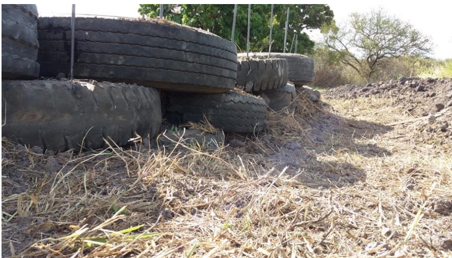
Figure 18 - Tire layout alternately. Source: Vasconcelos (2016).
