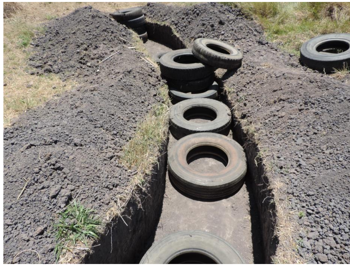
Figure 13 - Assembly of the first layer of tires. Source: Vasconcelos (2016).
