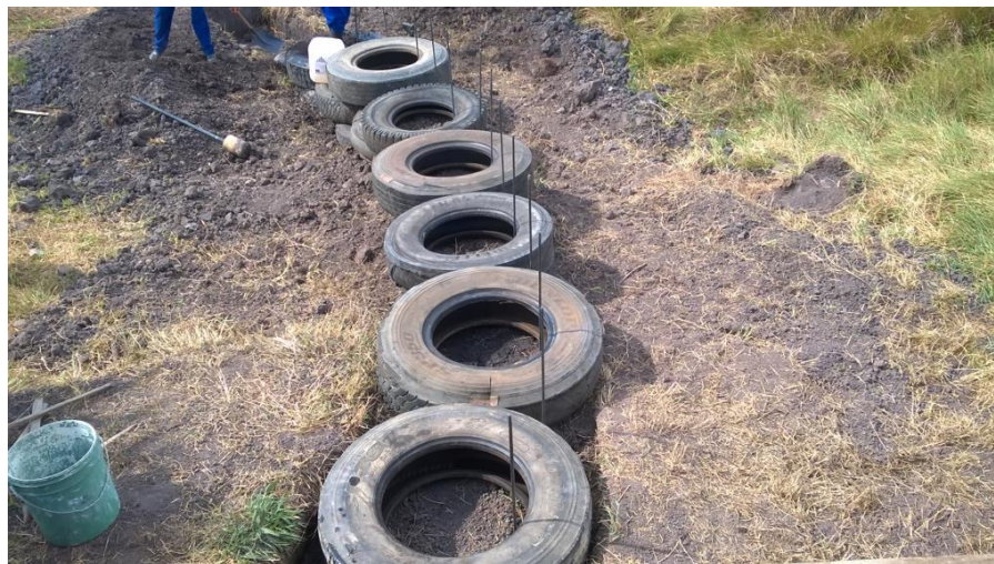
Figure 15 - Assembly of the third layer of tires. Source: Vasconcelos (2016).
