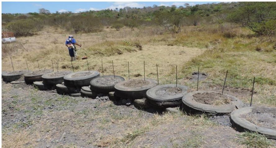
Figure 17 - Dam assembled with all layers and rods positioned. Source: Vasconcelos (2016).
