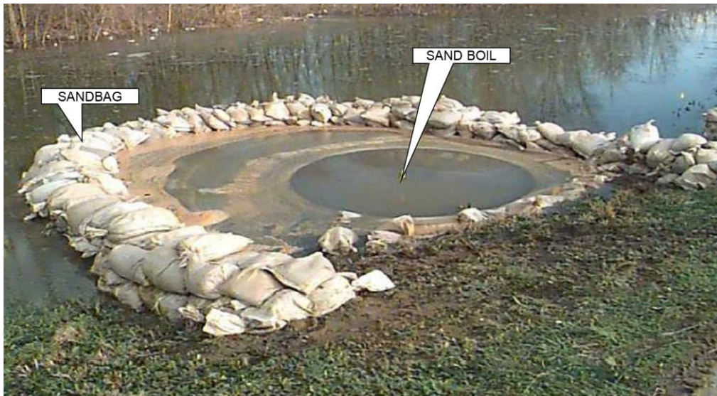
Figure 10. Sandbag Intercept Dike [FEMA] (2015).
