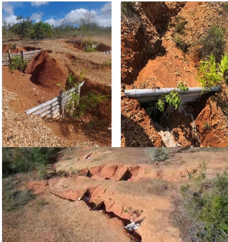
Figure 4. Ravines and check dams (palisades) located in plinthic soil in the municipality of São Cristóvão, Sergipe state, Brazil.
