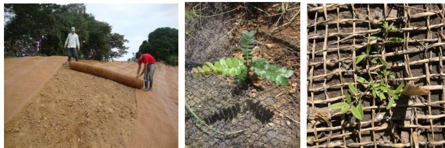
Figure 5. (a) Geotextile on the river slope, (b) synthetic geotextile, and (c) natural fiber geotextile in the municipality of Santana do São Francisco, Sergipe state, Brazil.
