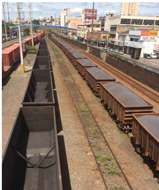
Figure 3: Railway transport system for the supply and disposal of steel production.
