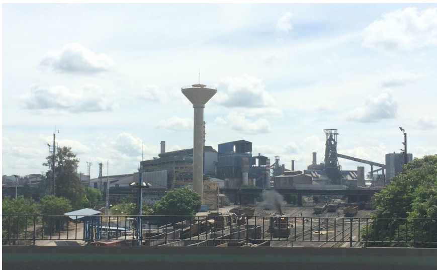
Figure 2: Presidente Vargas Steelworks (CSN) installations.
